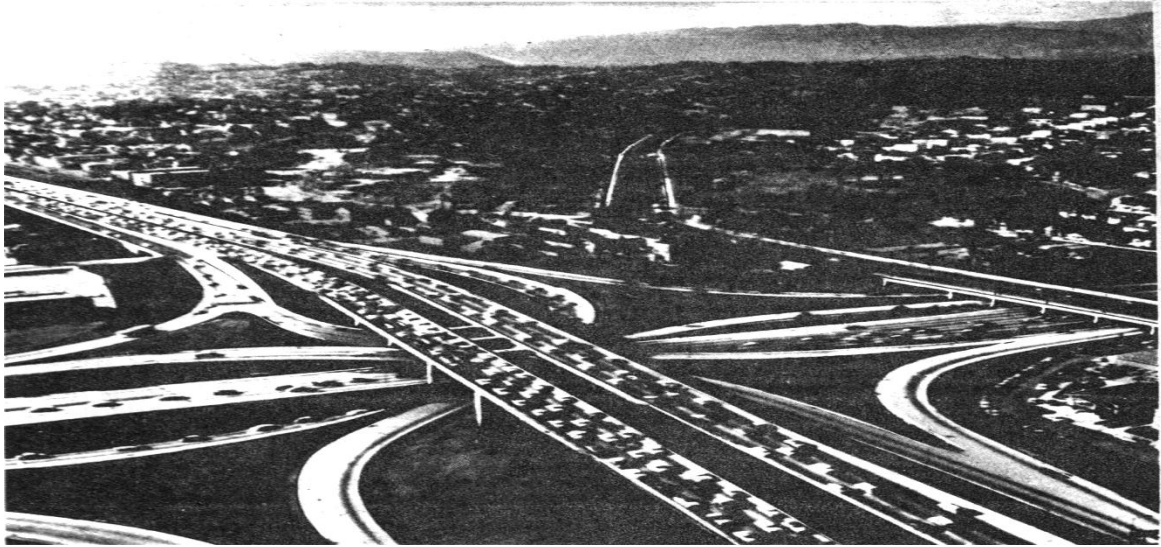
3.26-rasm. Chapga burilishli turdagi to'rt sathli kesishish.
