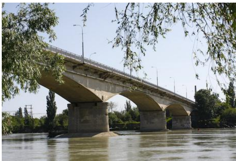
9.8-rasm. Katta temirbeton ko‘prik
