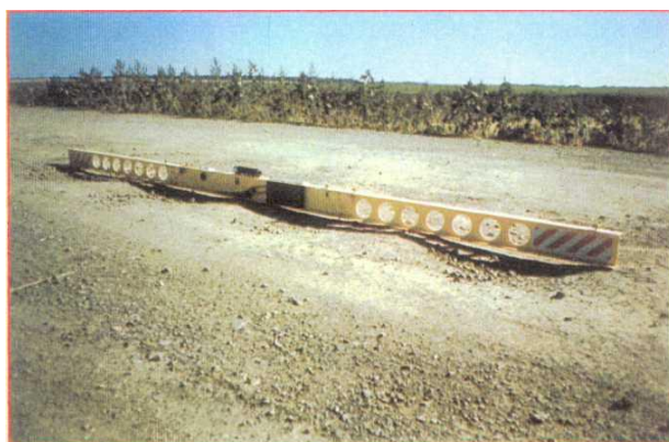
Rasm 6.5. Taroqsimon profil buzilishi
