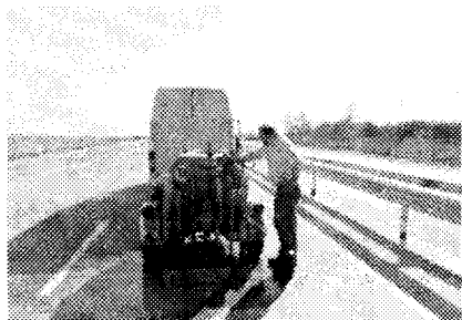
5.6-rasm. Qoplamadan diametri 15 sm o'lchamdagi silindrik kern namunasini burg'ulab olish jarayoni
