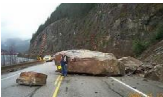
134-rasm. Ag'darmaning avtomobil yo'liga ta'siri
