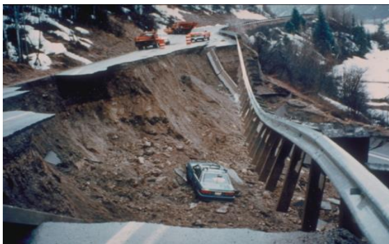
127-rasm. Ko'chki hodisasining avtomobil yo'liga ta'siri
