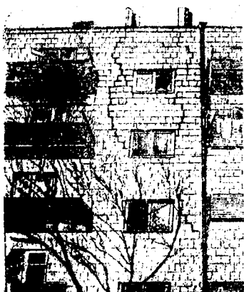
14.2-rasm. Zaminning o'ta cho'kishi natijasida yorilgan bino.
