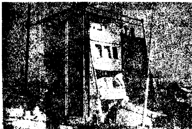
16.2-rasm. Zamin gruntlarining yuk ko'tarish qobiliyati susayishi natijasida cho'kkan bino (Armaniston. Spitak shahri).
