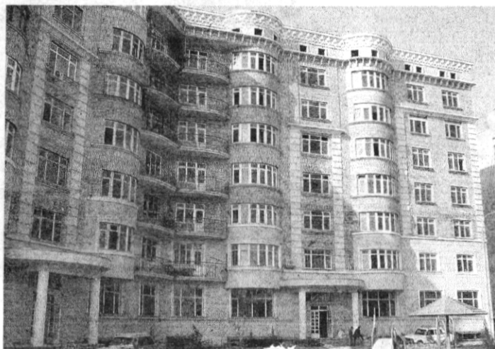
6.4-rasm. Toshkent shahridagi 7 qavatli zamonaviy turar-joy binosi
