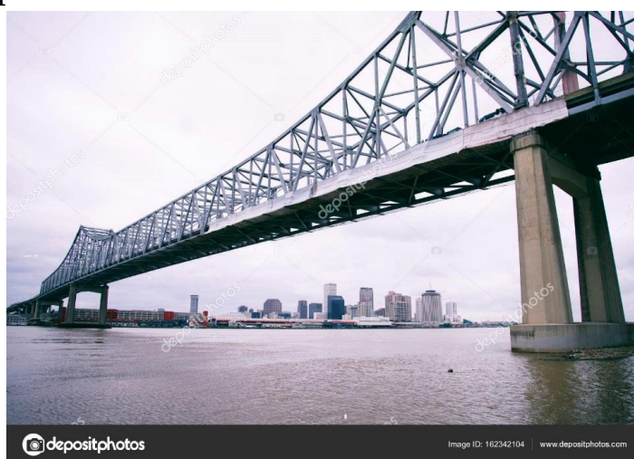
Rice. 1. Bridges with lattice trusses of large spans, USA
