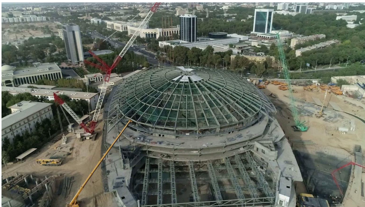
6.2-rasm. Humo arena muz saroyining aylana qovurg'ali gumbazi
