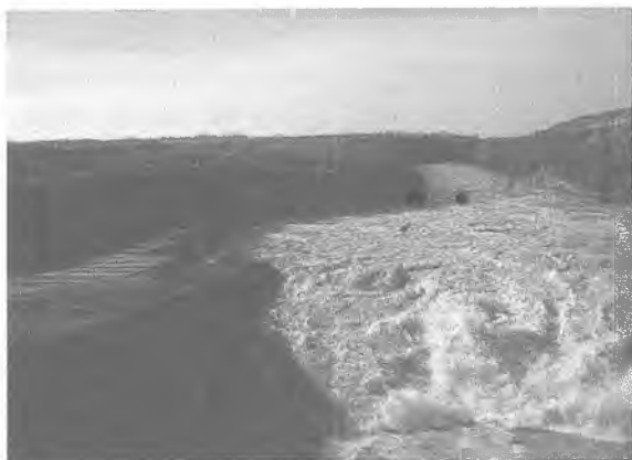
13.18 - rasm. Qiyshiq gidravlik sakrash oqibatida inshoot pastki befini yuvilishi.
