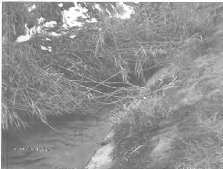
5.8 - rasm. Beton kanallar chetini o't bosishi
