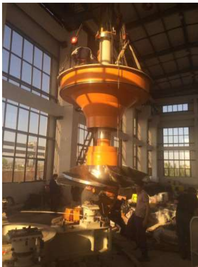
8.84-rasm. Mashina zalida burama kurakli turbinani o'rnatish
