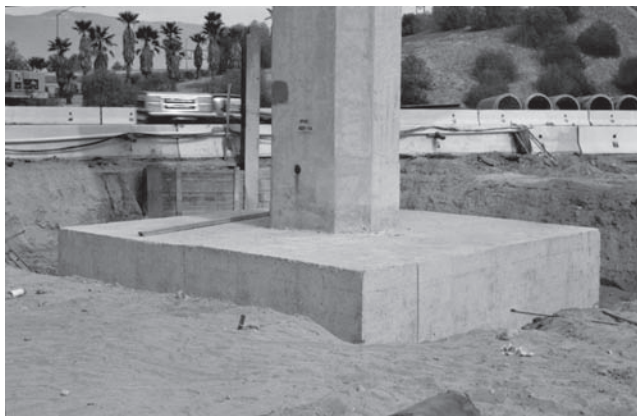
Figure 21.7 This bridge bent is supported on a group of pile foundations. The reinforced concrete cap connects the bent and the foundations. Because of the clean sandy soils at the site, this cap was cast using plywood forms which produced the smooth sides. However, in more cohesive soils, caps usually are cast directly against the soil.
