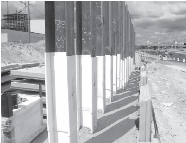
Figure 23.3 These H-piles will support a bridge abutment. They extend above the ground surface because the abutment fill has not yet been completed. Since the underlying soils are compressible and will settle due to the weight of the fill, the piles have been wrapped with a specially designed lubricated plastic sheeting to reduce the downdrag forces between the piles and the fill. A mechanically stabilized earth (MSE) wall is being constructed around these piles. When complete, the backfill will extend approximately 1 m above the wrapped area of the piles (courtesy of Foundation Technologies Inc.).
