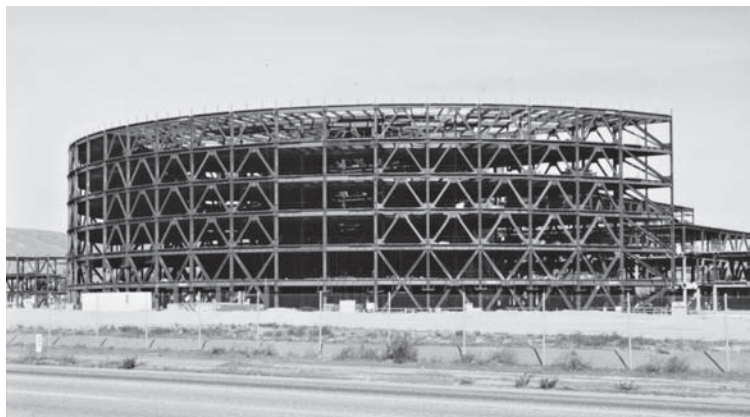
Figure 8.13 The diagonal bracing in this steel-frame structure has been installed to resist seismic loads. However, a side benefit is that this bracing provides more rigidity, which helps even out potential differential settlements. Shear walls have a similar effect. The two bays in the center of the photograph have no diagonal bracing, and thus would be more susceptible to differential settlement problems.
