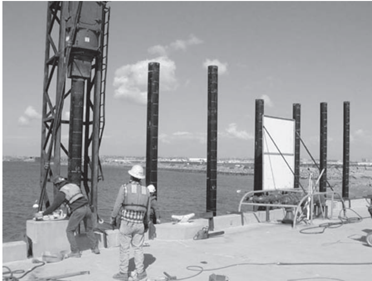
Figure 12.15 Installation of plastic-steel composite piles in a waterfront application (photo courtesy of Lancaster Composites, Inc.).
