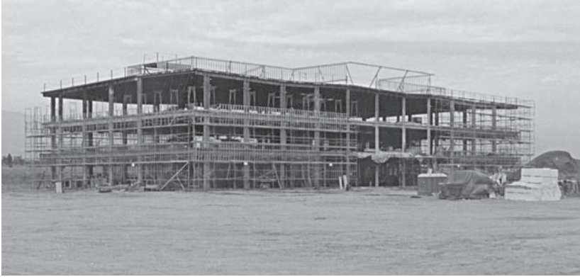
Figure 8.12 This steel-frame structure has no diagonal bracing or shear walls, and thus would be classified as “flexible.”
