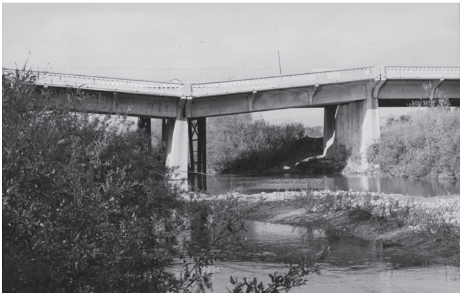
Figure 9.15 One of the mid-channel piers supporting this bridge sank about 1.5 m when it was undermined by scour in the river channel.
