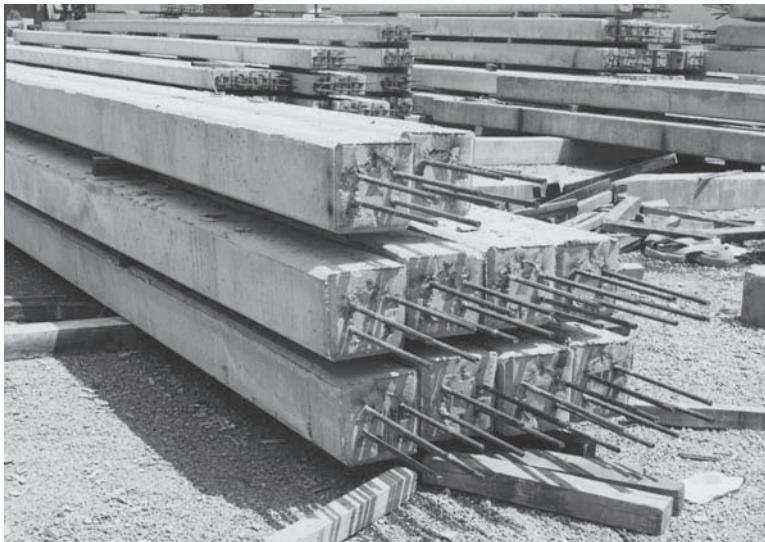
Figure 12.11 These 356 mm (14 in) square prestressed concrete piles are stacked in a contractor's yard and are ready to be driven. The bars emerging from the end of these piles are conventional rebars that have been embedded in the end of the pile (they are not the reinforcing tendons). These rebars are used to structurally connect the pile with the pile cap.
