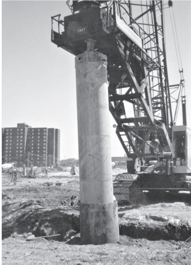
Figure 12.39 The contractor at this site is using casing. The first casing, visible at the bottom of the photography, is already in place. However, its length is limited by the height of the rig. When casing must extend to greater depths, a second smaller casing is installed by passing it through the first casing, as shown here.
