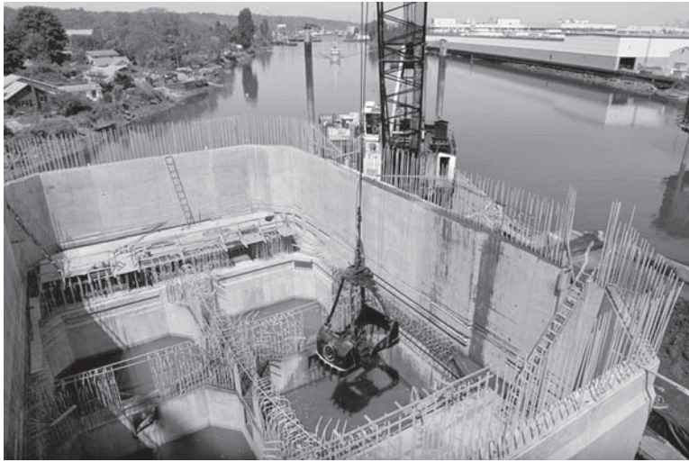
Figure 12.58 An open caisson being dredged. The walls of this caisson are cast in place and raised as the caisson is cut into the river bed (photo by John Stamets).
