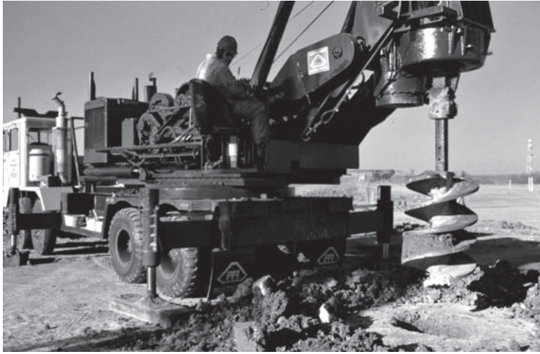
Figure 12.32 Typical flight auger (ADSC: The International Association of Foundation Drilling).
