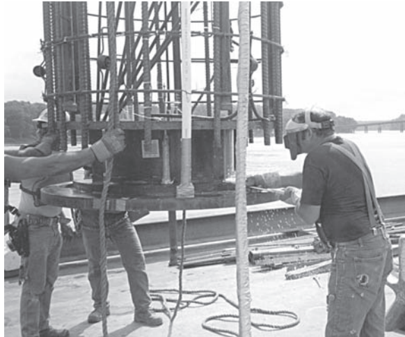
Figure 14.13 An Osterberg cell being installed at the bottom of a drilled shaft rebar cage (Loadtest, Inc.).
