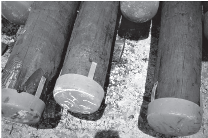
Figure 12.5 Use of steel toe points to reduce damage to timber piles during driving (Associated Pile and Fitting Corp.).
