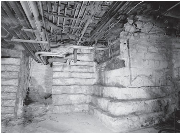
Figure 6.4 Dimensional stone foundation for Chicago Auditorium building built between 1887–89. Note both height and width of the foundation and the amount of space they occupy. (Library of Congress, Prints & Photographs Division, HABS, Reproduction number HABS ILL, 16-CHIG, 39-8.)
