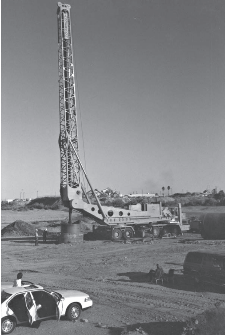
Figure 12.31 Extremely large drill rig capable of drilling 8 m (26 ft) diameter holes to depths of 60 m (200 ft) (courtesy of Hayward Baker Inc.).
