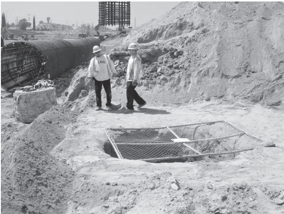
Figure 23.9 This 2.4 m (8 ft) diameter drilled shaft will support a bridge bent. It has been excavated using the dry method and the steel reinforcing cage is about to be placed. Another similar steel cage is visible in the background. The chain-like fencing is a safety precaution and is about to be removed.
