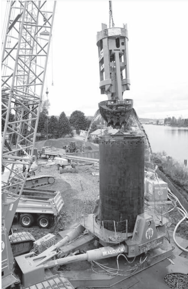
Figure 12.40 The casing for this large-diameter drilled shaft was installed by a device known as an oscillator. The oscillator is the steel table-like device holding the casing at the ground surface. The oscillator rotates the casing back and forth using the hydraulic ram attached in a vee pattern. It also provides a downward thrust on the casing. The oscillating motion and the downward thrust force the casing into the ground. The bottom of the casing is fitted with teeth to aid it in penetrating the ground. In this particular project, the shaft is being excavated with a hammer grab, which is a heavy bucket-type device that opens into a circular shape. It is dropped quickly into the shaft to break up the soil at the bottom of the shaft. When it is retracted the grab closes and removes the loosened soil (photo by John Stamets).
