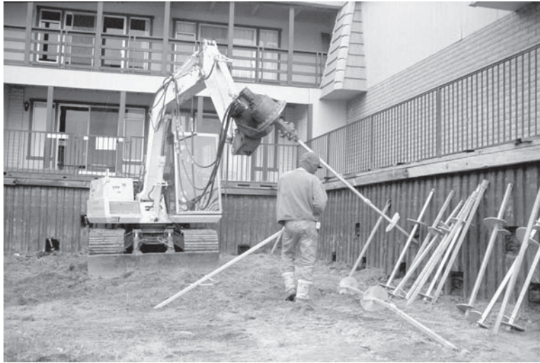
Figure 12.56 Installation of a helical anchor to be used as a tieback for a sheet pile wall. Once these anchors are installed, the soil in the foreground will be excavated (photo courtesy of A. B. Chance Company).
