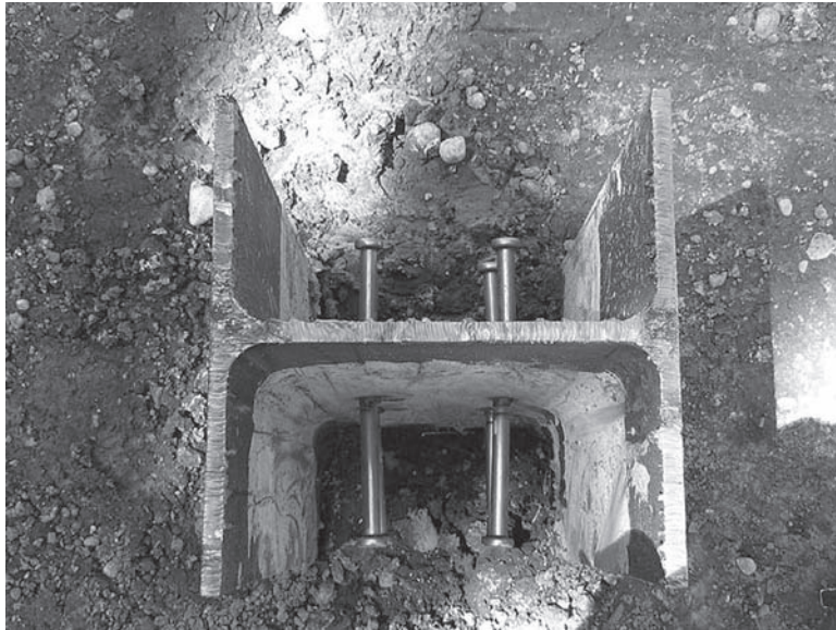
Figure 12.6 A steel H-pile after being driven in the ground. The nail-like items welded on the pile web are shear studs which help to secure the pile in the concrete pile cap that will be cast around the pile. Note that the web and flange of the H-pile are the same thickness, unlike a WF section whose flange is thicker than its web. Source: King County Dept of Transportation.
