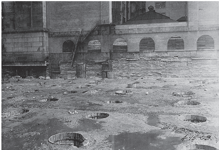
Figure 12.27 Shaft excavations for Chicago City Hall made in 1909 using the Chicago Well Method. The wooden shoring for each shaft is clearly visible. These shafts were dug by hand down to the desired foundation depth (Library of Congress, Prints and Photographs Division, Historic American Buildings Survey, HABS ILL,16-CHIG,94-36).
