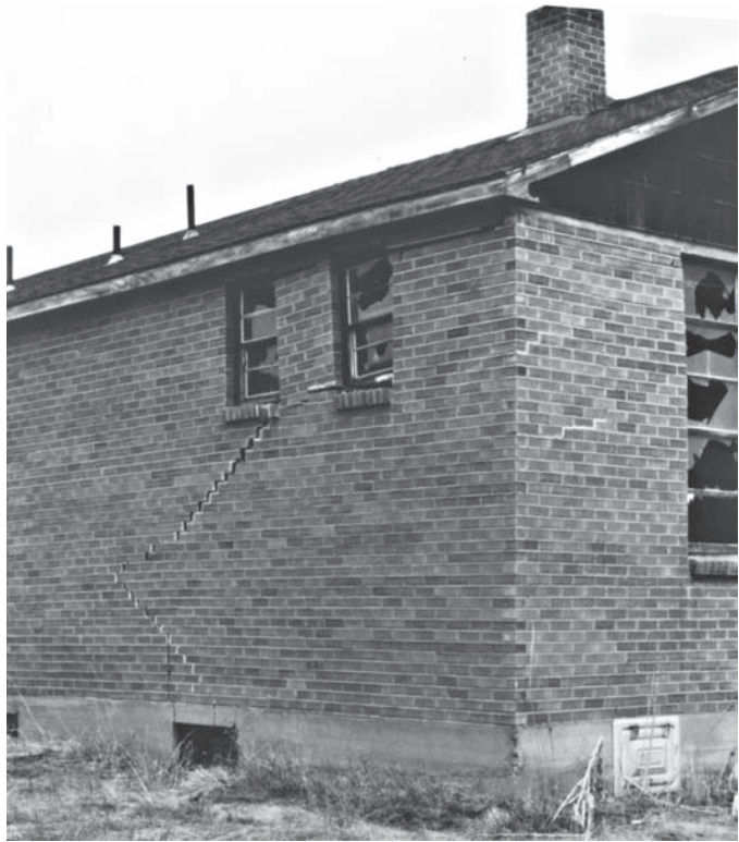
Figure 27.3 Expansive soils caused this brick building to crack (photo courtesy of the Colorado Geological Survey).
