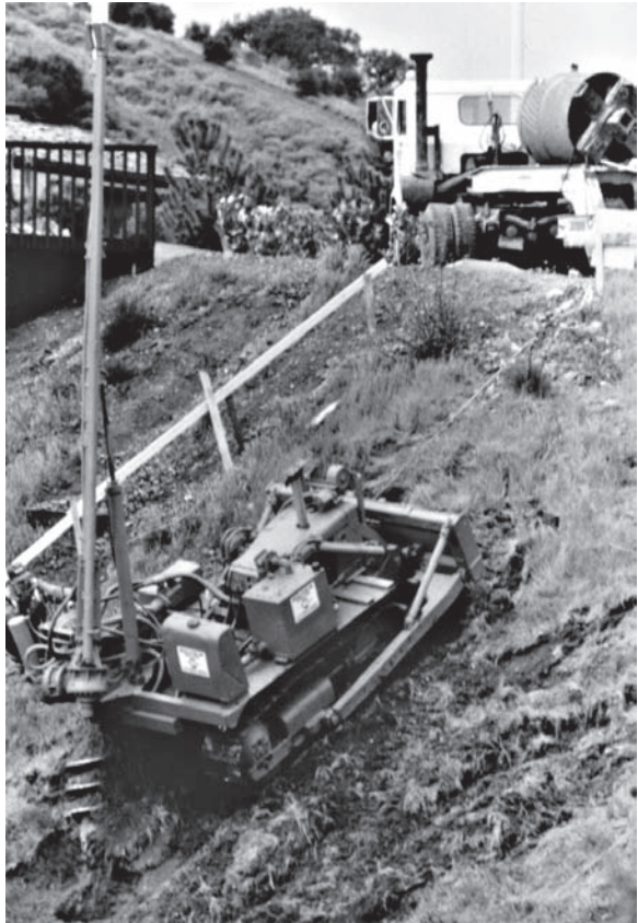
Figure 12.30 Small truck-mounted drilling rig capable of working on a hillside (ADSC: The International Association of Foundation Drilling).
