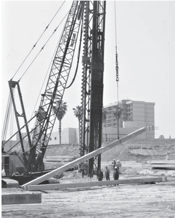
Figure 21.1 This prestressed concrete pile is being lifted into the pile leads by a single cable. This process induces handling stresses in the pile.
