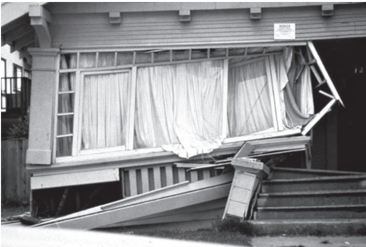
Figure 10.29 House that separated from its foundation during the 1989 Loma Prieta Earthquake (photo by C. Stover, U.S. Geological Survey).
