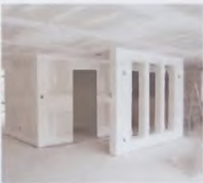
44-rasm. Gipsokarton list GKLO
