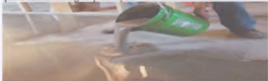
72-rasm. Polimer betondan pol quyish jarayoni
