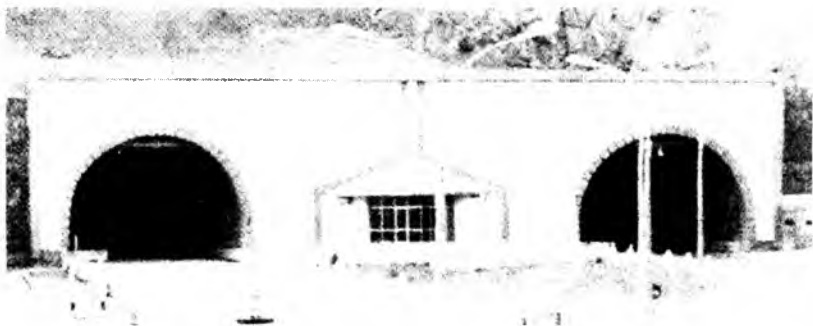
13.8-rasm. Qamchiq dovonidagi tunellarning kirish joyi
