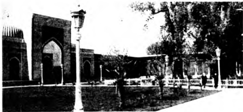
13.24-rasm. Samarqand. Imom al-Buxoriy majmuasidagi masjid (chapda)
