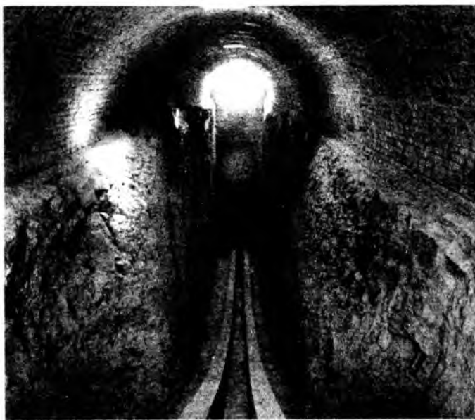
9.32-rasm. Ulug'bek rasadxonasining burchak o'lchagichi
