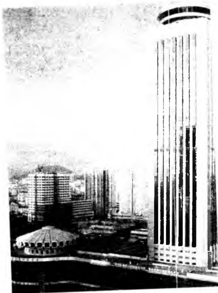
7.39-rasm. Shanxay shahridagi zamonaviy osmono'par binolar
