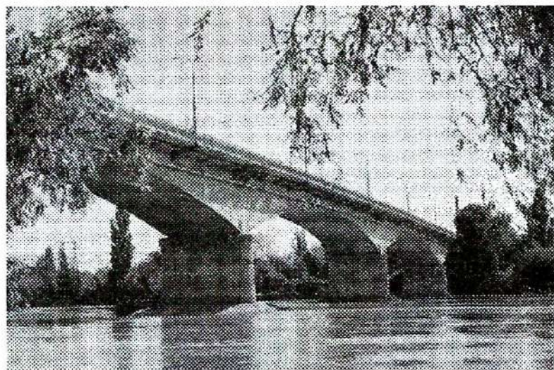
9.8-rasm. Katta temirbeton ko'prik
