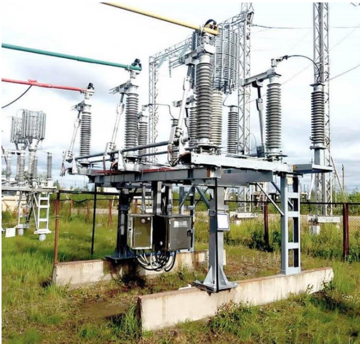
4.6-rasm. RLND-2-110/600 markali ajratgich.
