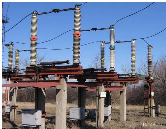
6.13-rasm. ОД-110/600 markali bo'lgich: 1 – yuritma, 2 – richaglar tizimi, 3 – izolyatsion tayanch, 4 – chiqish kontaktlari, 5 – yumshoq ulanish, 6 – kontakt pichoqlari, 7 – kontakt lamellari, 8 – himoya qobig'i, 9 – fundament.
