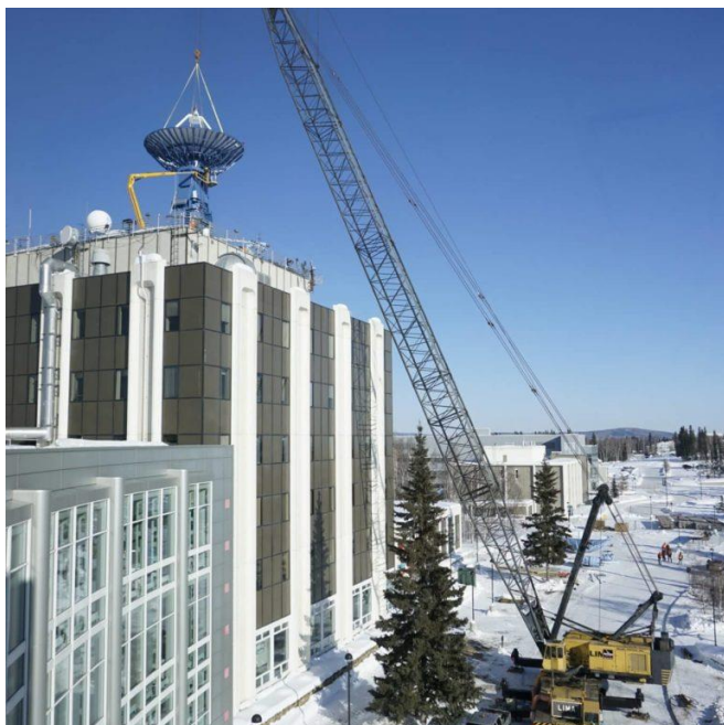
5.6-rasm. AS2 antenasining almashtirilishi. (manba https://asf.alaska.edu/timeline/ )
