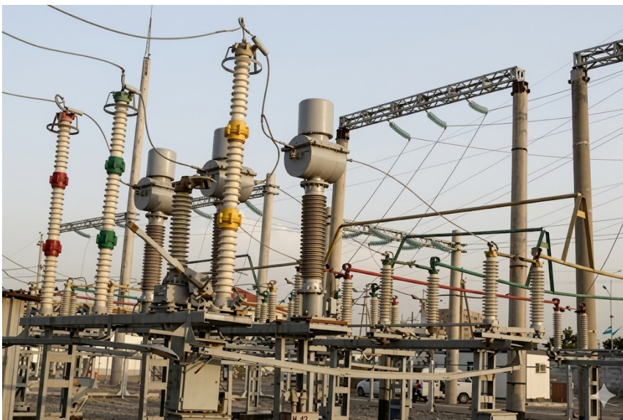
2-rasm. Podstansiya elektr jihozlarini o‘ta kuchlanishdan himoyalashda razryadlagichlar ko‘rinishi
