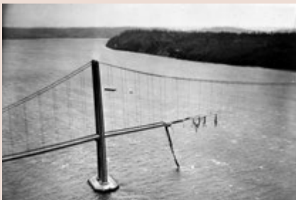
Collapse of the Tacoma Narrows Bridge
